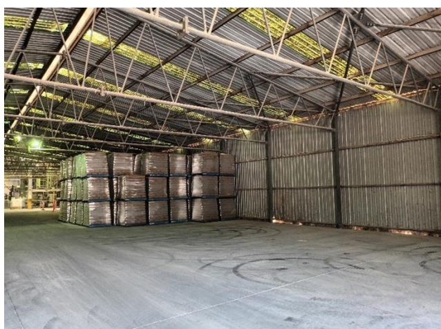
Geraldton Industrial Property – warehouse space
